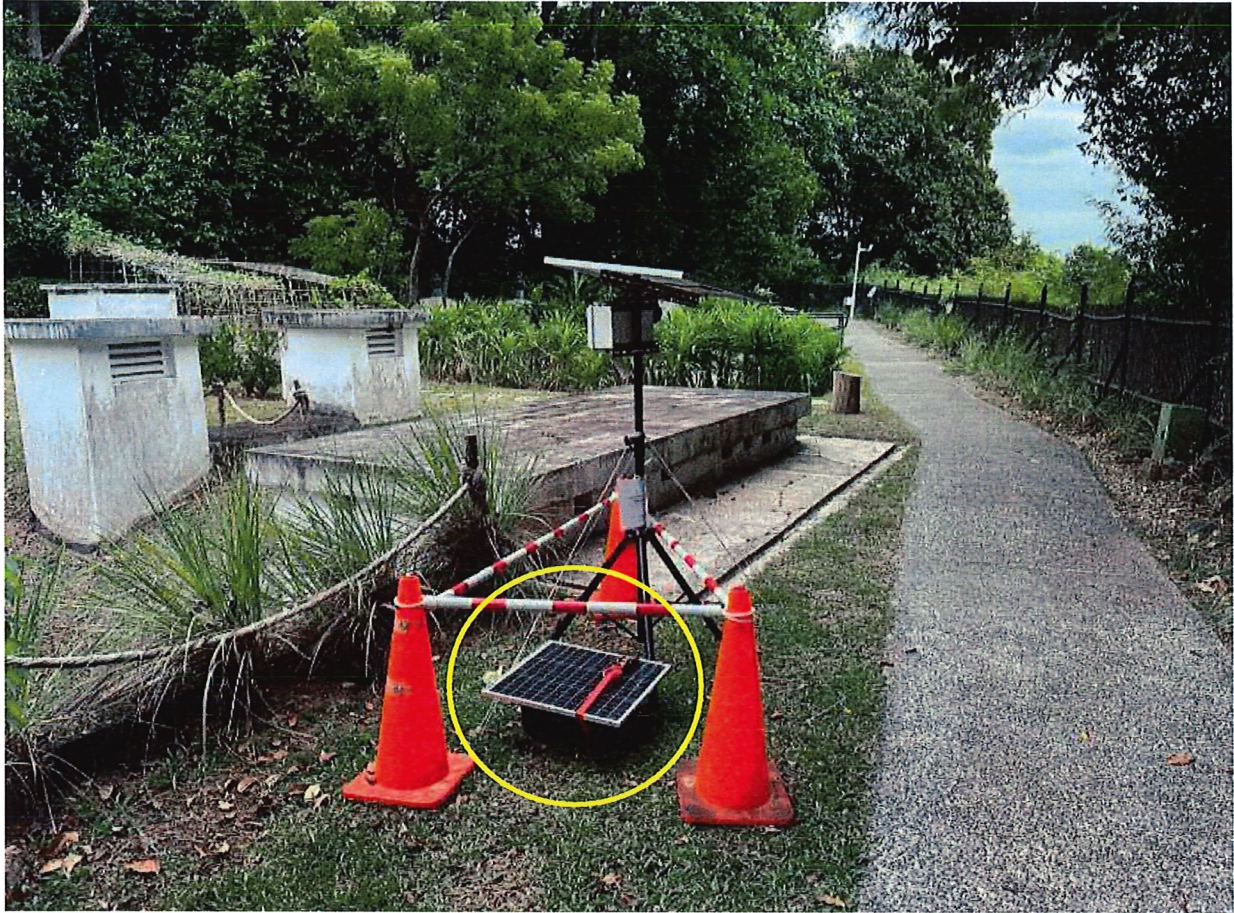
Photos: Vibration Monitoring Station at V1 (16/10/2025)
